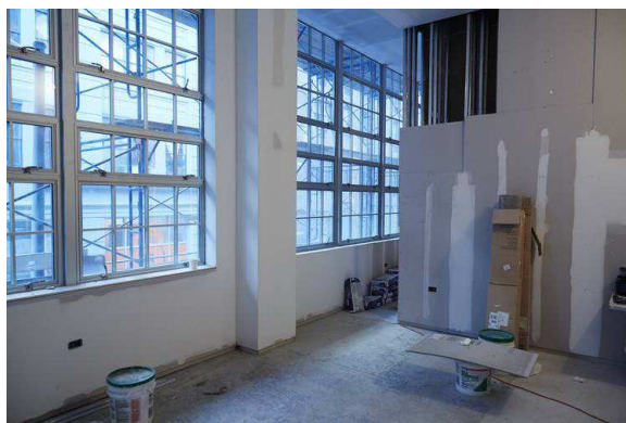
The former factory windows have been enlarged for use by condo residents.
